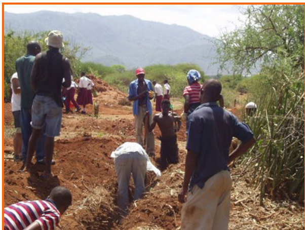
Foundations for schoolroom, Mwanga, Northern Tanzania, November 2007
